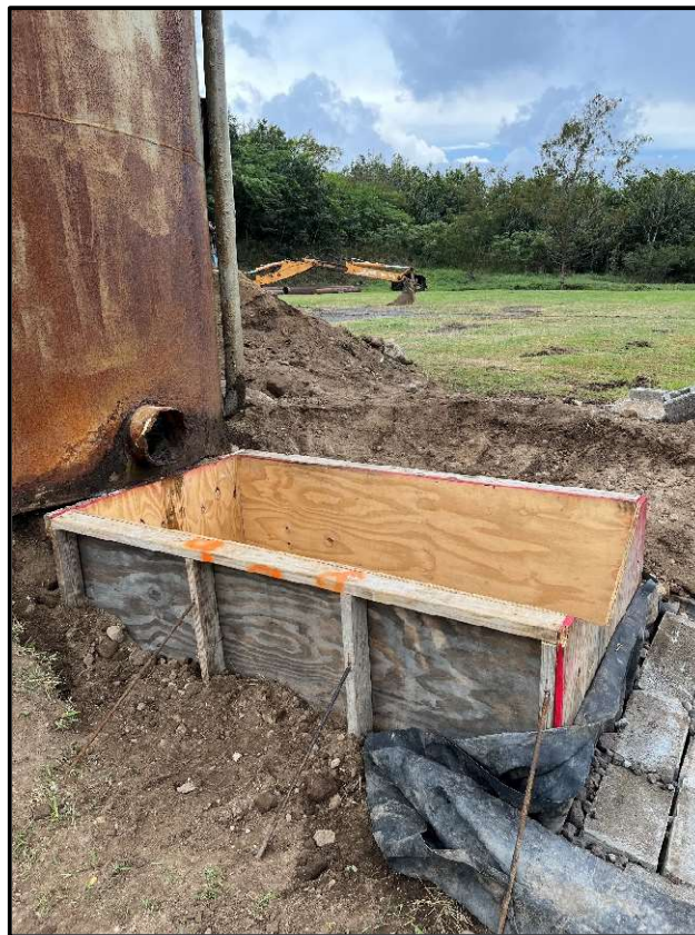
Figure 16: Weir box set up in place on outlet of separator. The weir box measured 79" x 40" x 40" with a 120 degree V-notch weir extending to each side with the point of the V-notch 29" up from the bottom
