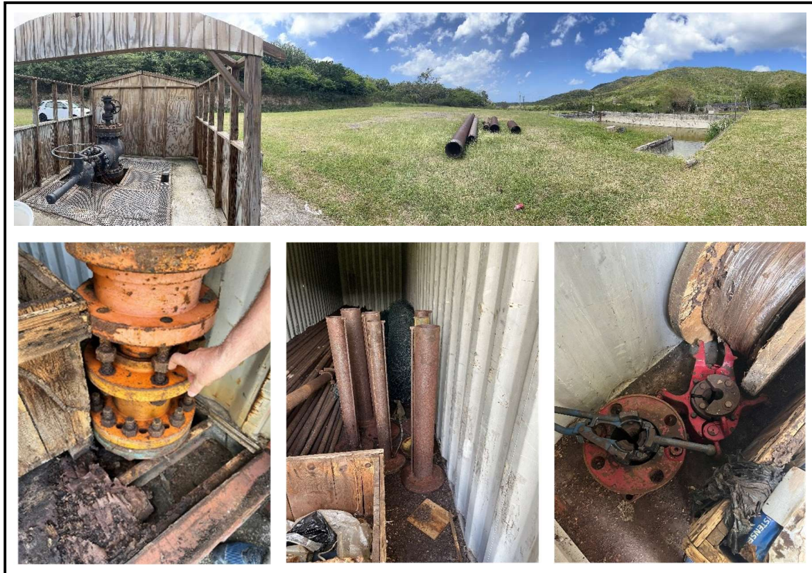
Figure 3: Pictures above show the initial condition of the MON-2 well site (top) along with the initial condition of the Giberson head (bottom left), the James Tubes (bottom centre), the slips, elevators and spare 0.092" Wire (bottom right).
