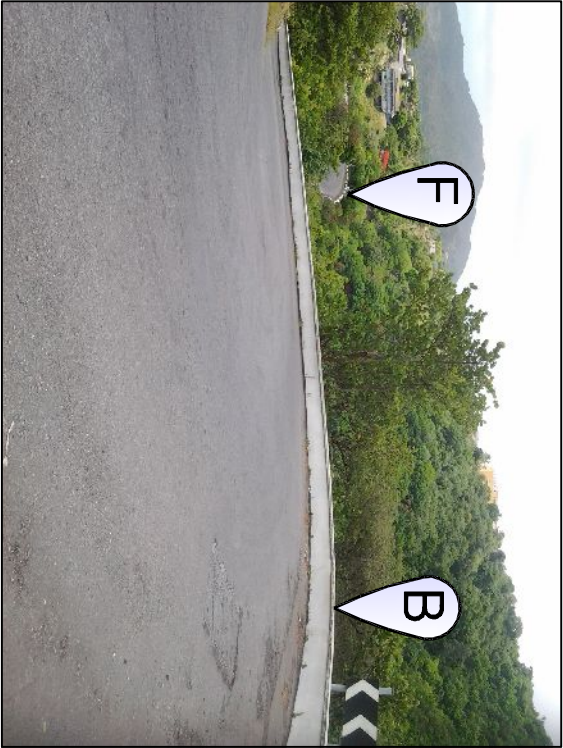
B) Concrete Headwall- 173'-0"L x 26"H
