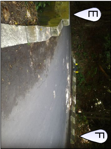
D Concrete Headwall- - 173'-0"L x 30"H
