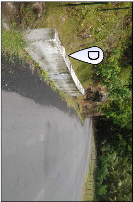
D Concrete Headwall- - 173'-0"L x 30"H
