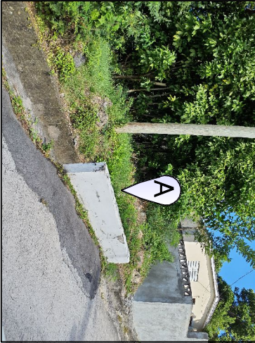
A Concrete Headwall 9'-0"L x 24"H
