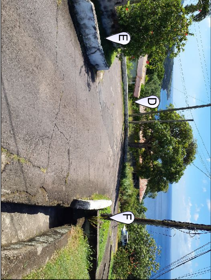
D Concrete Headwall- 64'-0" L x 20" H
