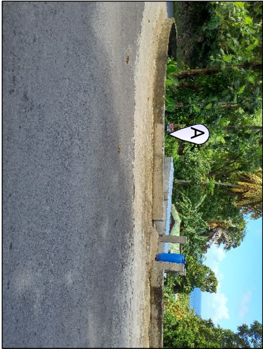
A Concrete Headwall 124'-0" L x 24" H
