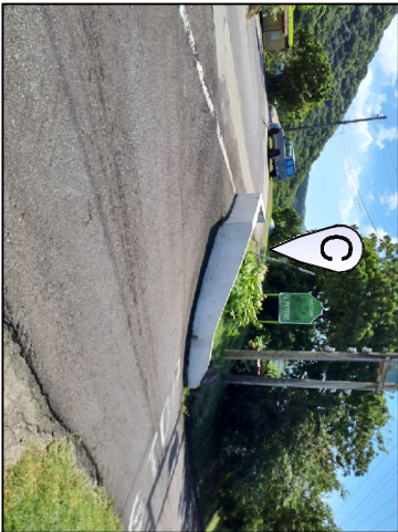
C Concrete Headwall 27'-0"L x 20"H
