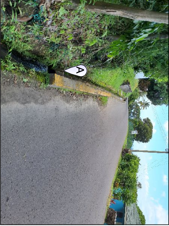
A Concrete Headwall 27'-0" L x 16" H
