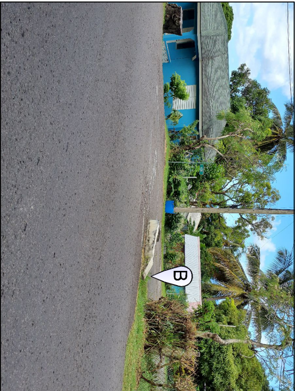
B Concrete Headwall 11'-0" L x 16" H
