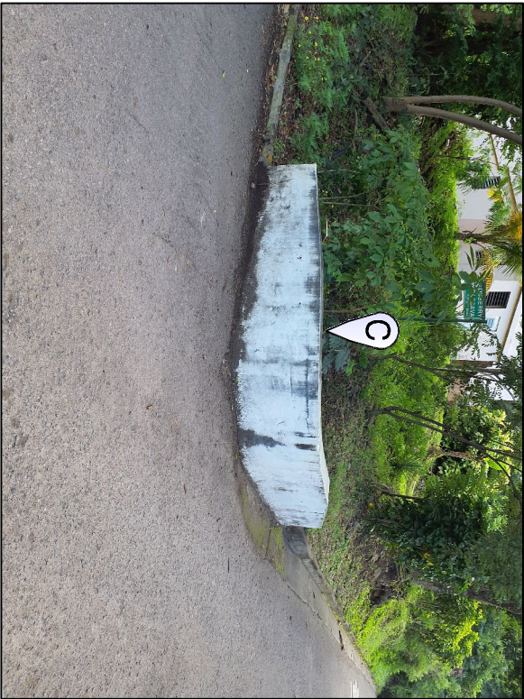
C Concrete Headwall 16'-0" L x 24" H
